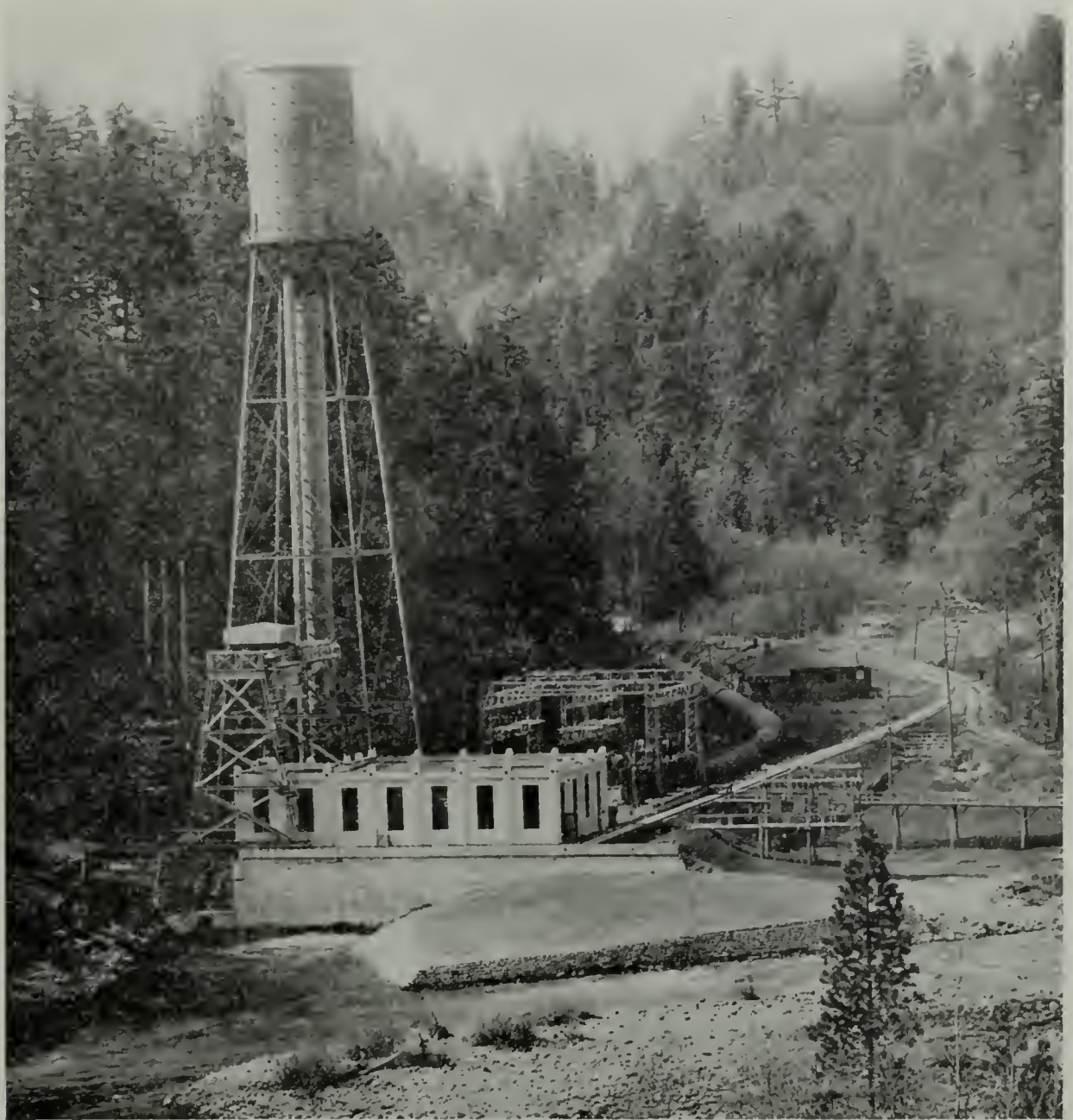
Powerdale Generating Station - constructed in 1922 by Pacific Power & Light Company.
